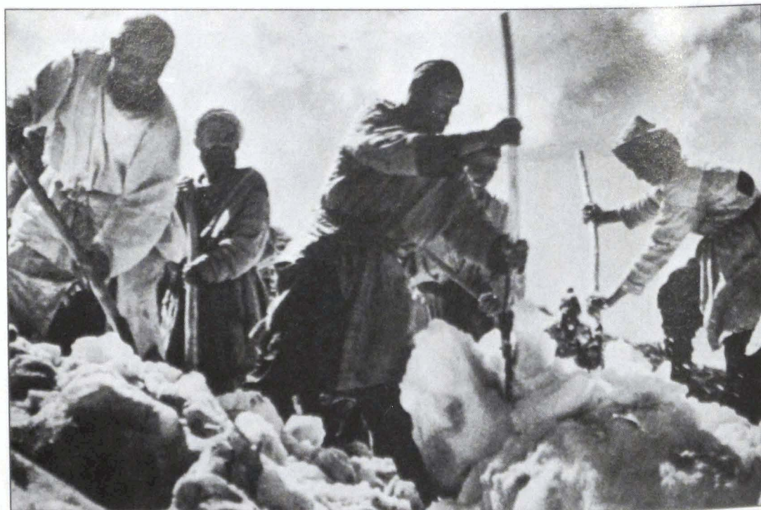
15. Blasting the Osh–Khurug road, 1940s
