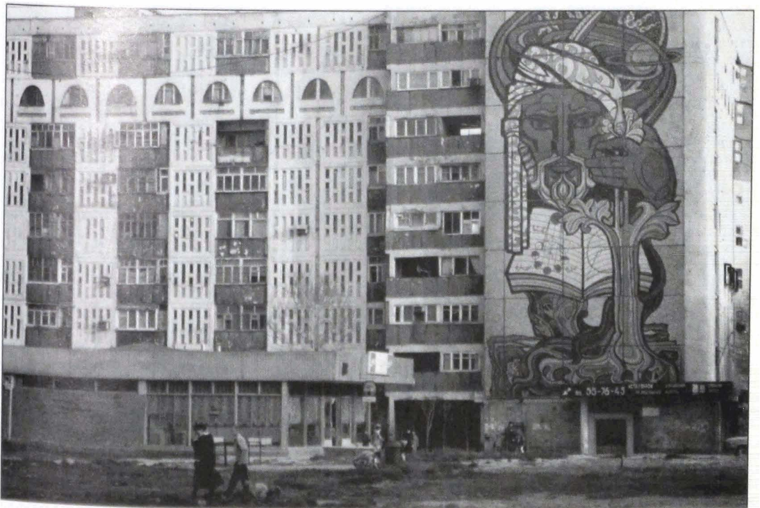
29. Soviet-era flats, Tashkent: domestic architecture was given an eastern flavour by the inclusion of characteristic closed balconies derived from the classical avivan . The mural is of Ibn Sina
